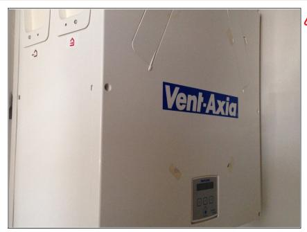
Turn the heat recovery system off at the wall.
